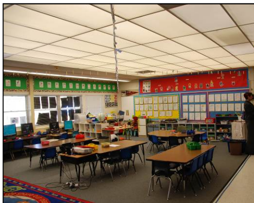
Classrooms are generally in good condition. Some finishes & new ceiling lenses needed
