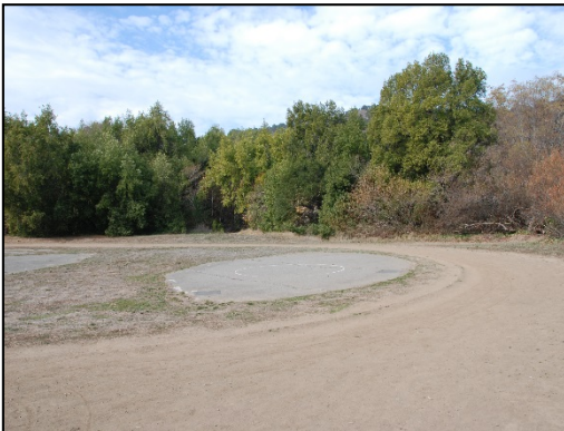
West-side track in extremely poor
