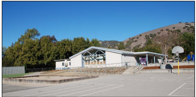
Option to add additional kindergarten south of K-2 including new retaining wall & replacement ramp
