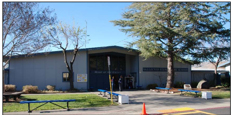
Administration entry difficult to find and lobby small. Expand lobby into staff room and provide pergola or other element to create strong sense of campus entry.
