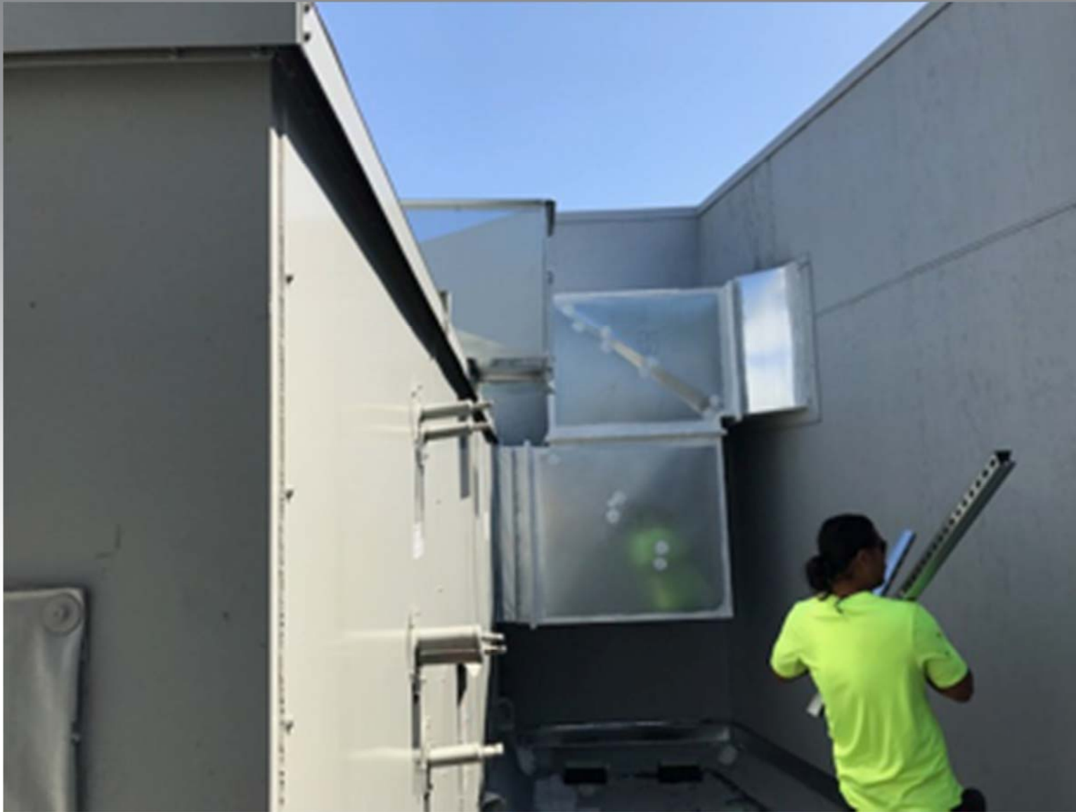
Supply ductwork installed onto AHU-1
