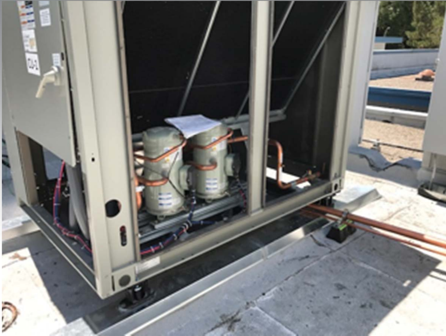
New condenser unit installed
